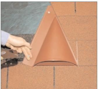
Ventilating your roof will equalize the temperature of the outer and inner roof. Your roof structure will then be able to withstand sudden temperature changes.
